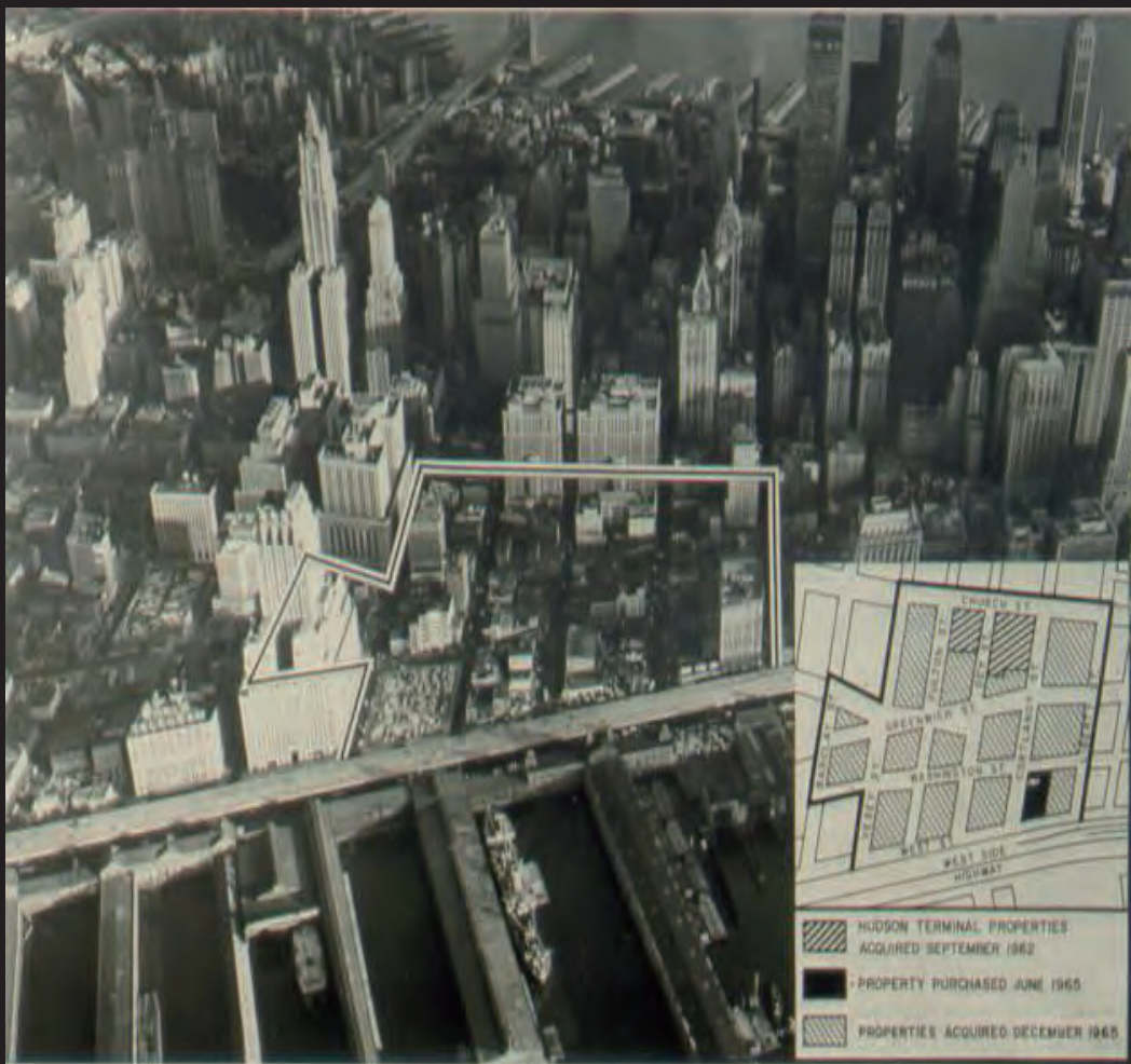
SITE OF WORLD TRADE CENTER TO BE BUILT BY THE PORT OF NEW YORK AUTHORITY IN LOWER MANHATTAN
